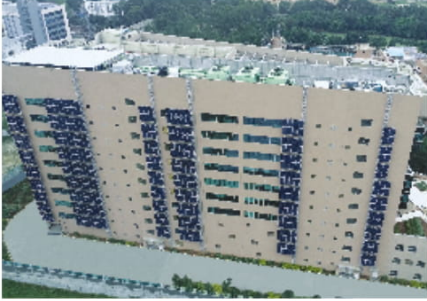
Building Integrated PV Dell International, Bengaluru
