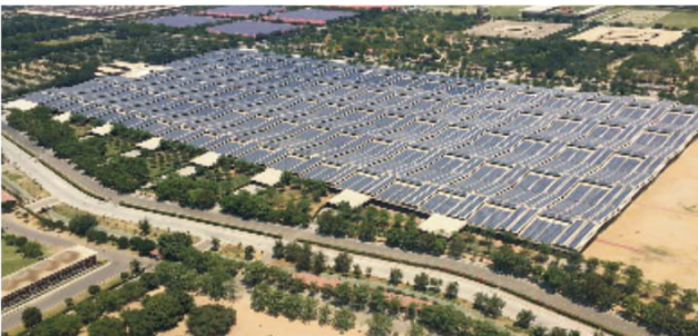
World's Largest 16 MW Rooftop Solar Plant at R.S.S.B. Educational & Environmental Society (RSSB-EES)
